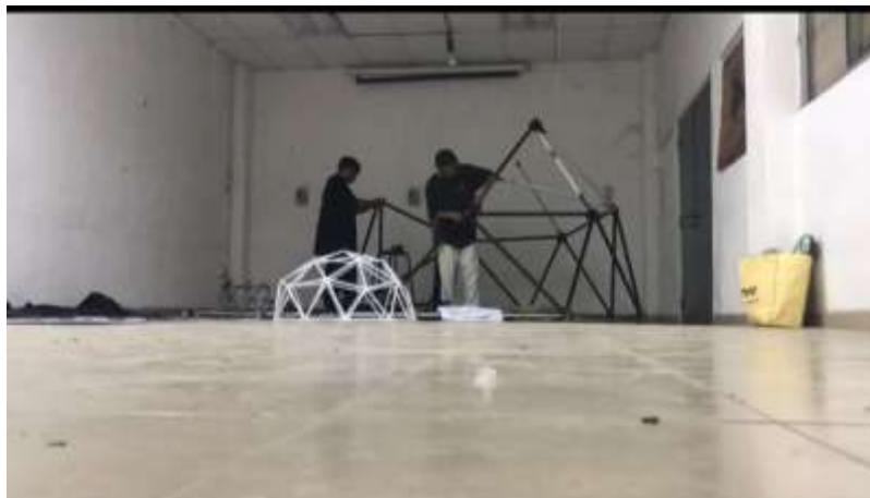
Picture 5 : Installation of the dome
